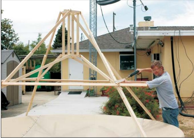
Figure 8 · Construction of the feed support structure.
